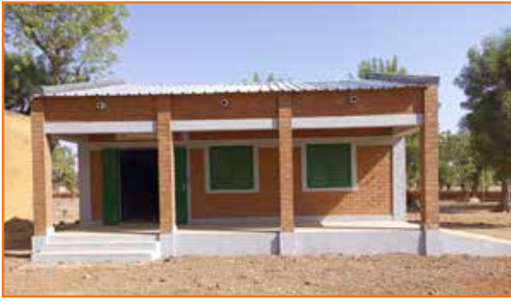
Tanguin school classroom building cofunded by the Foundation
