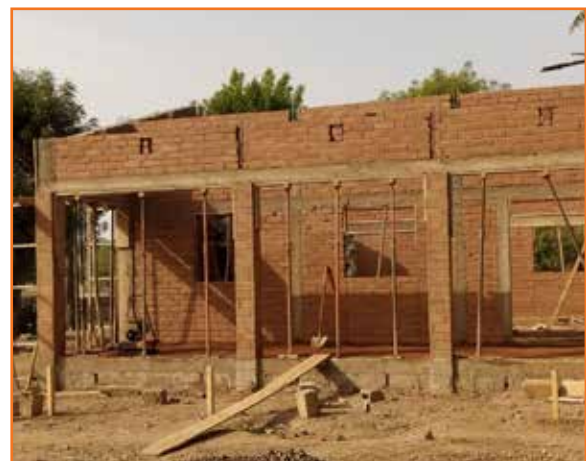
School building in construction
