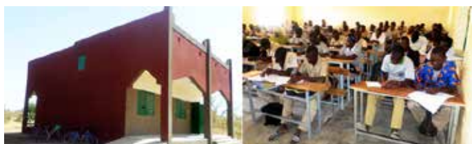
New Classroom at Sogpelce' Secondary School Campus built in 2015
