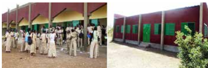
Sogpelce' Secondary School and Library Building built by the Foundation
